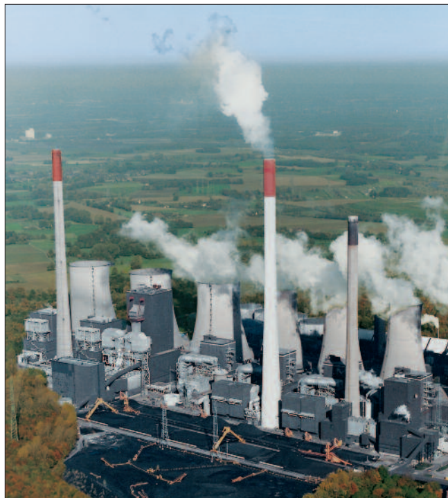
Power plant (EON)
