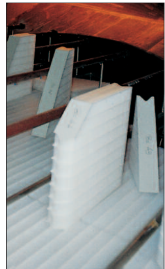
LTV 271 during installation
