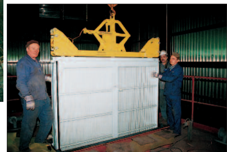
LTH 100 being installed in a flue-gas desulphurization plant
